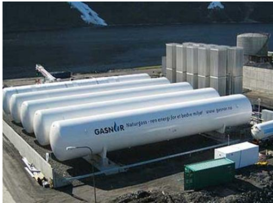
Figure 11. Example of semi-pressurized tanks
