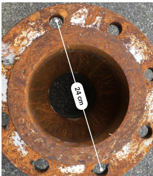
Flange 4. DN 150, 6 inch – 8 holes
